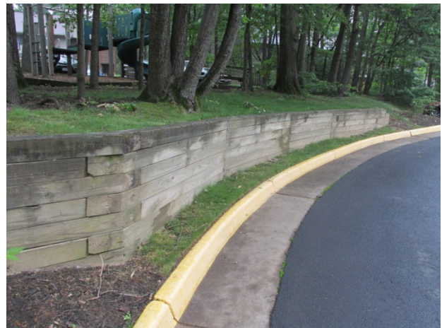
Retaining wall overview
