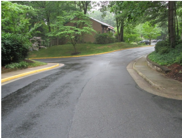
Asphalt pavement overview
