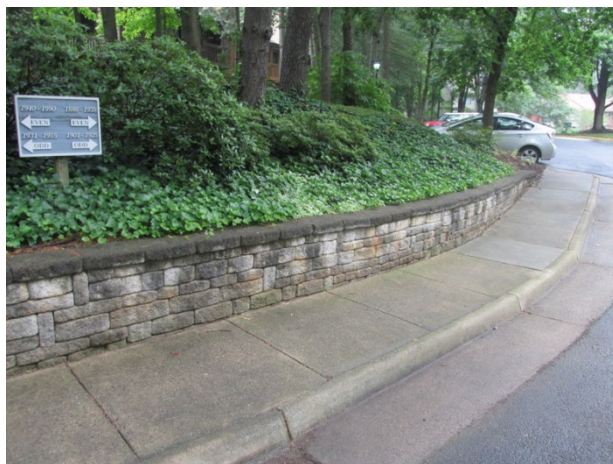
Masonry retaining wall overview
