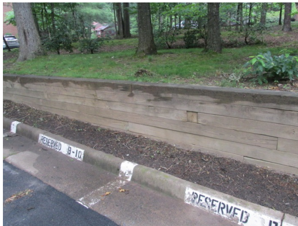
Timber retaining wall overview
