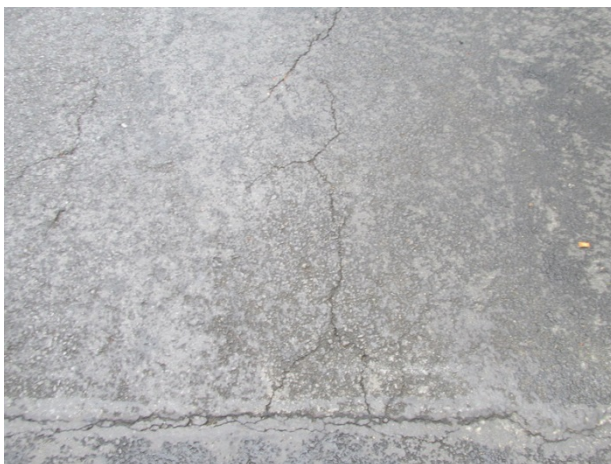
Pavement cracks
